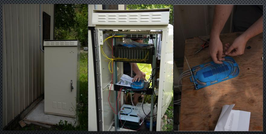
This is where fibre cables are spliced to individual fibre connectors on an **Optical Distribution** Frame and then connected to Switch Ports. Main line fibres are 10 Gbps and service fibres are 1 Gbps at the Switch 144 circuits served but with room for 72 more
